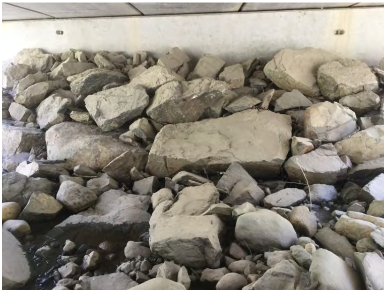
Right Bank Abutment when facing downstream
