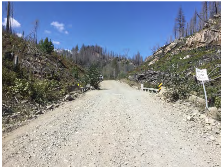
Approach from Right Bank when facing downstream
