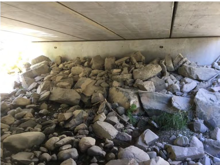
Left Bank Abutment when facing downstream
